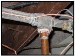
Copper/Galvanized piping contact is noted. Correction is recommended (4C.o6).
