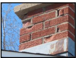
Chimney shows evidence of spalling - surface deterioration of the bricks. This condition should be monitored because if spalling continues, rebuilding the chimney will ultimately be necessary (1B.02).
