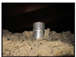
Bathroom vent should not discharge into the attic (8C.16, 9D & 3C.12).
