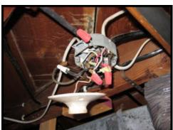
Hanging light fixture in basement needs to be secured. NOTE: The current electrical box may be exceeding the cable fill requirements. Please have an electrician verify this during the repair.
