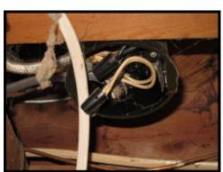
All junction boxes should be fitted with cover plates, in order to protect the wire connections (5C.06).
