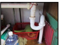
An S Trap has been used. Ideally, S traps should be replaced as they are subject to siphoning problems. S traps are common in older homes. Replacement is sometimes difficult and thus the S traps are usually tolerated. Care should be taken to keep the trap primed. Fixtures should be monitored for sewer odor (4A.08).
